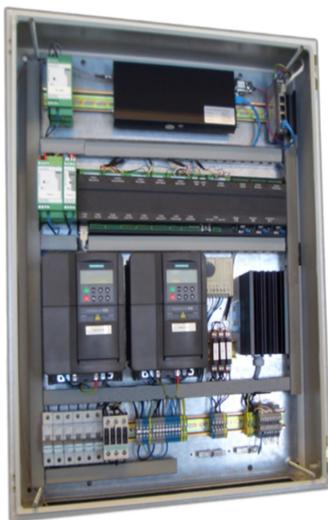
The DIN Rail Module can be directly integrated into a cabinet at the antenna. Together with the **sat-nms** LBRX Beacon Receiver, also available as DIN Rail Module, it is possible to have a complete step-track system integrated into the antenna cabinet.
