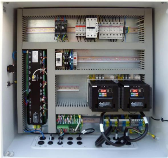
*ACU-ODU-AC-DE, standard with 4kW inverters*
