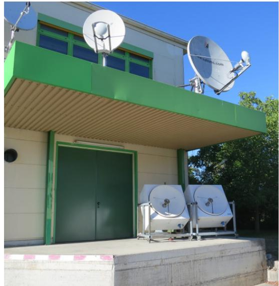
SatService GmbH has two own radiometers for operation at 14.7GHz. These two radiometers were manufactured in 1988 by the company Elektronikcentralen. SatService GmbH retrofitted and upgraded the radiometers with the **sat-nms** RMC radiometer controller, **sat-nms** RMD Radiometer Detector and an electrical motorization in elevation axis. These Radiometers could be rented.
