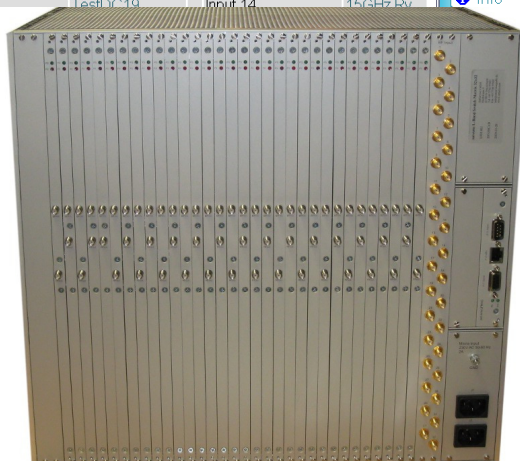
Rear View of 32x32 Matrix Crosspoints
